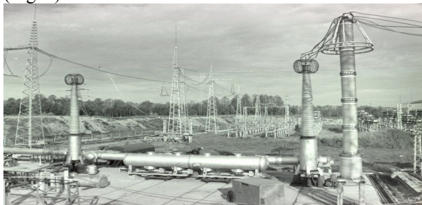
Fig. 1 1150 kV gas insulated switchgear (GIS) at Togliatti Power Testing Laboratory, Russia, 1979.
