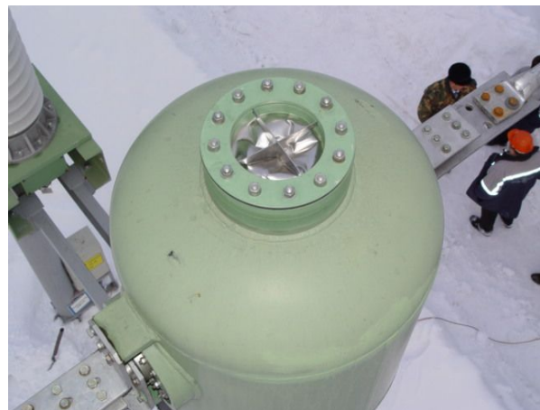
Fig. 3 Defect of the instrument current transformer - the break of the membrane.
