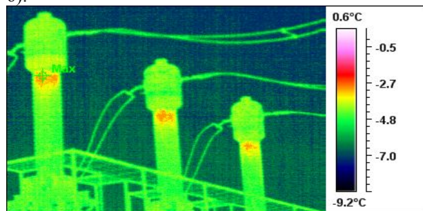
Fig. 6 Heat-gram of SF6 insulation current transformer ( \Delta T=2,1 oC).
