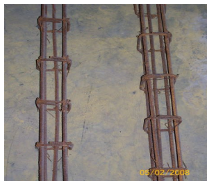
Fig.3.1 Steel Reinforcements
