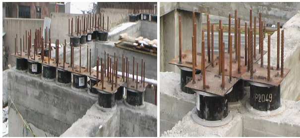
Fig. 5. Examples on installation of rubber bearings' clusters in the 15-story base isolated apartment building "Avan"
