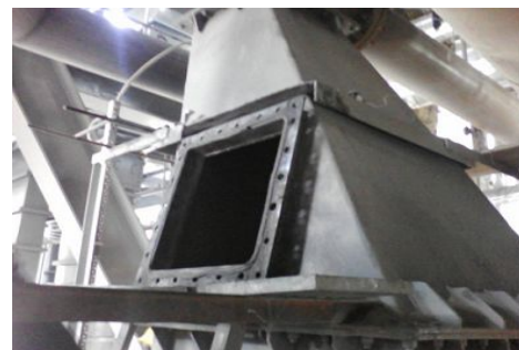
Photo 1 – Manhole details in bed ash cooler
