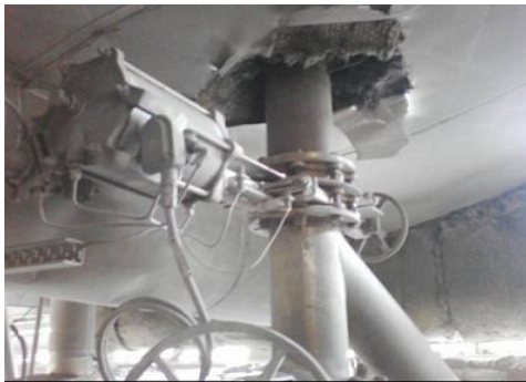
Photo 3 – Pneumatic slide gate in hot ash entry to ash cooler
