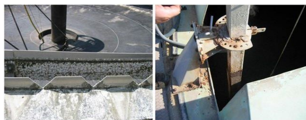
Figure 7: (left) pitting in decanter (stell surface) and (right) electrochemical corrosion in metallic elements (authors).
