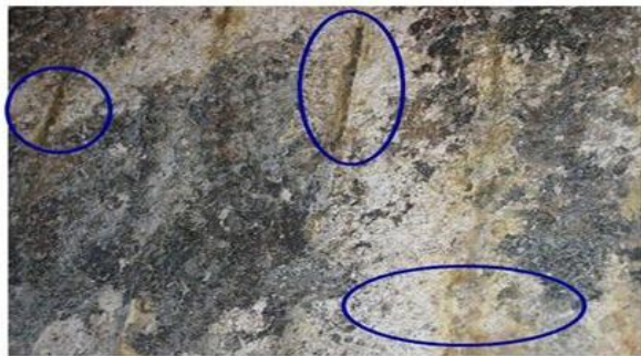
Figure 2: Corrosion by sulfurs in internal walls of wastewater collector (authors).
