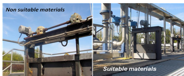
Figure 9: Application of non-suitable and suitable materials in WWTP elements (authors).
