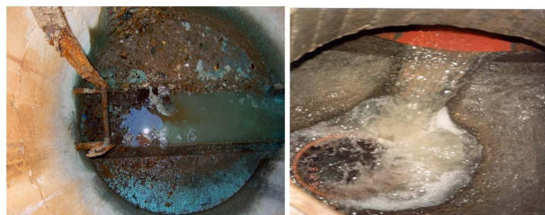
Figure 6: (left) chemical acidic corrosion and (right) chemical alkaline corrosion in industrial wastewater rush to general network (authors).
