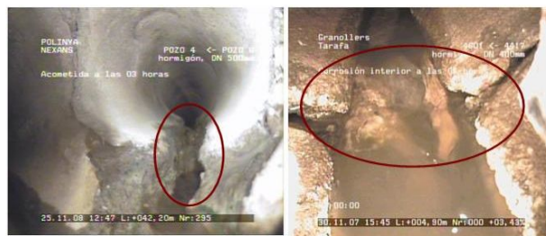
Figure 5: Chemical corrosion on two high diameter wastewater collectors (authors).
