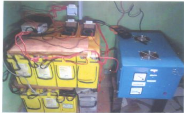
Appendix 2: The Twenty (20) Solar Panels of 80W, 12V each
