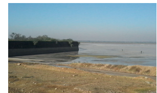
Fig-4: Water supply channels
