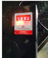
Fig: III – Battery Charger
