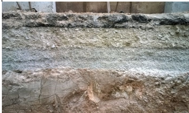
Fig 3: Pavement excavation showing layers
