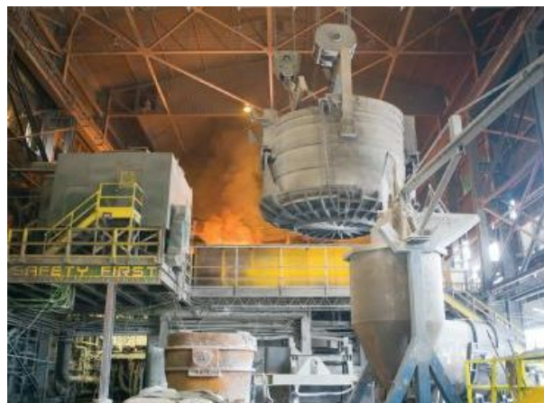
Fig3 Lifting of tarpedo car with the help of cranes
