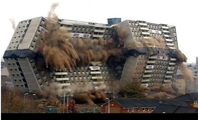
Fig 6. Demolition of building by explosion (falling into footprint)
