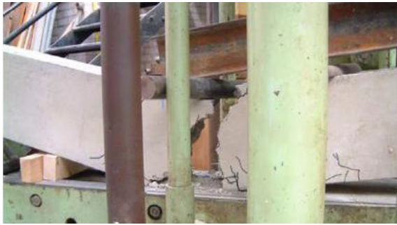
Fig.: Flexural failure of specimen
