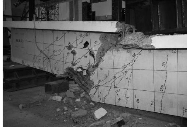
Fig: Shear failure of test specimen (E.A. Ahmed et al 2008) [6]
