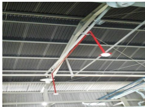
Figure 4. Light bulbs in PLTMG-CNG Bawean.
