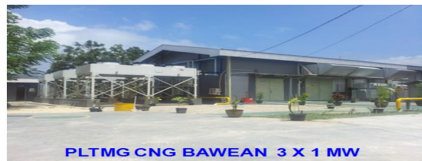
Figure 1. PLTMG-CNG Bawean site view.
