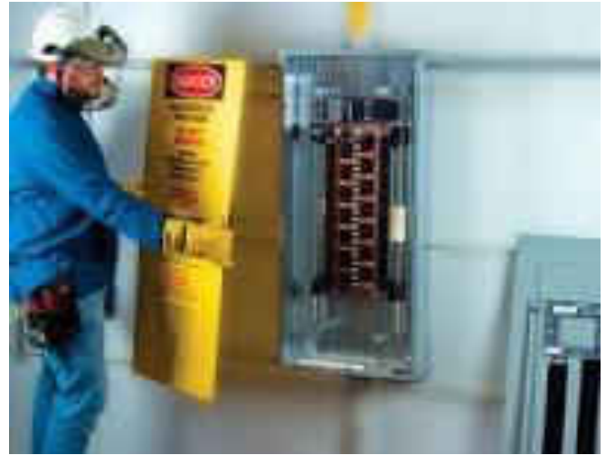
Electrical wiring with proper safety equipments in a developed nation
