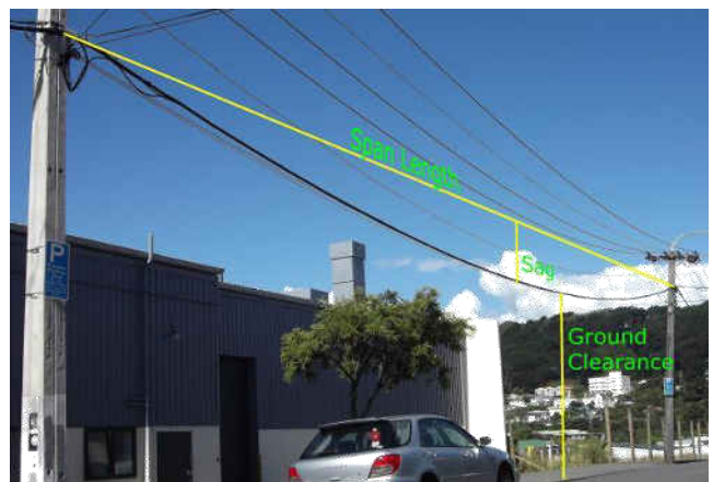
Hanging wires with sufficient ground clearance
