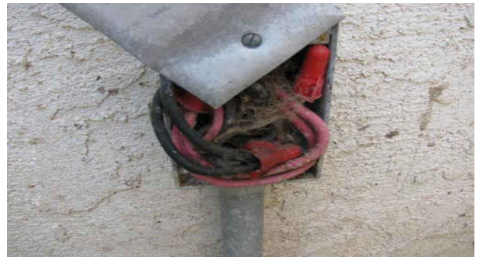
Wires left hanging after renovation
