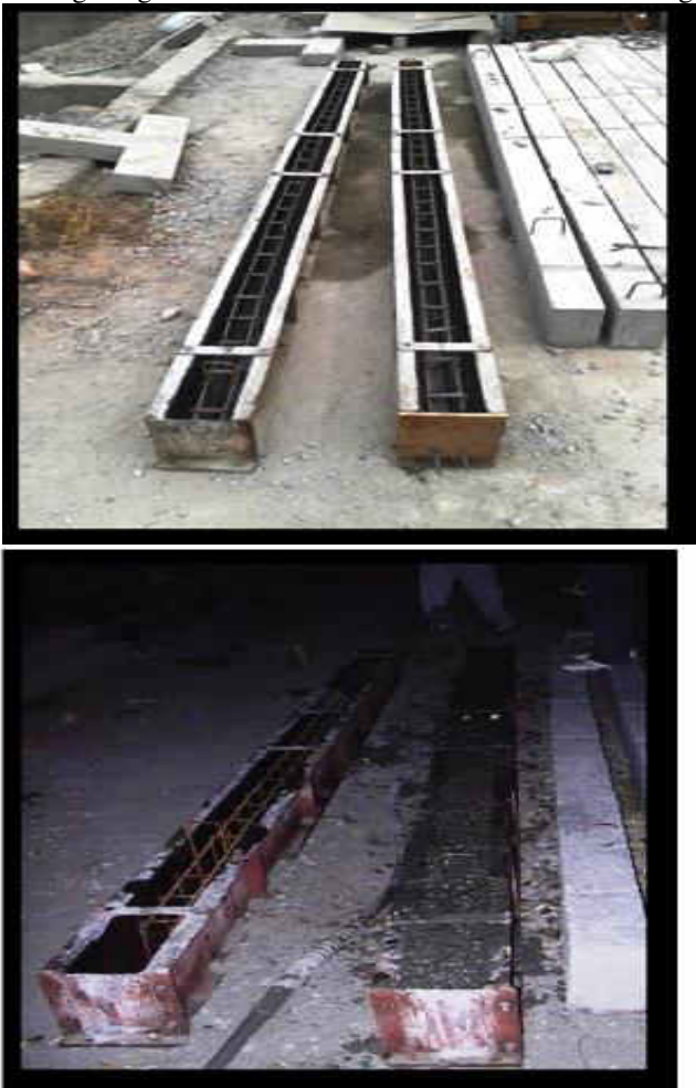
Fig. 3.2 Beams Before and After Casting Mass Loss Determination
