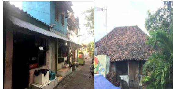
Figure 2. Condition of houses Gubeng Kertajaya 2
