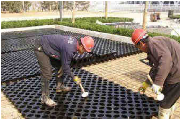
Fig.2 Formwork Arrangement Construction
