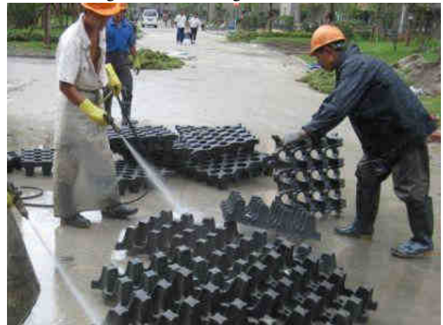
Fig. 3 Formwork cleaning
