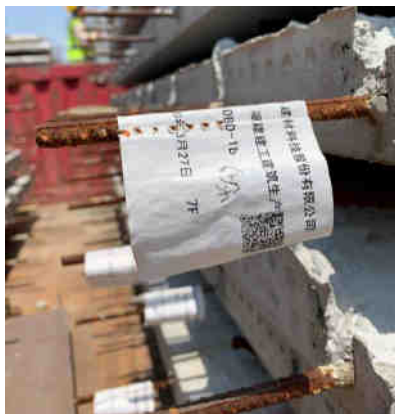
Fig. 6 Component identification
