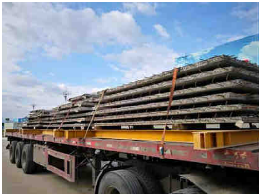
Fig. 5 Production and transportation of prefabricated components
