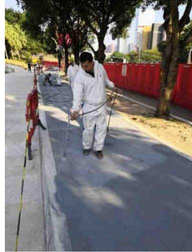
Fig.4 Spray sealant
