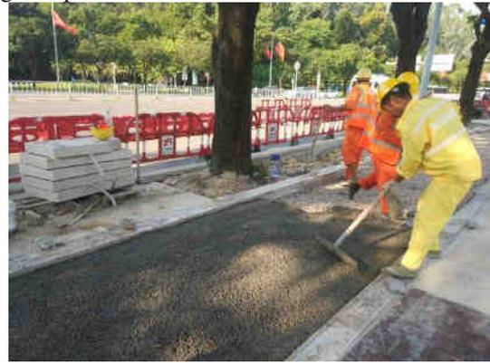
Fig.1 Permeable concrete paving
