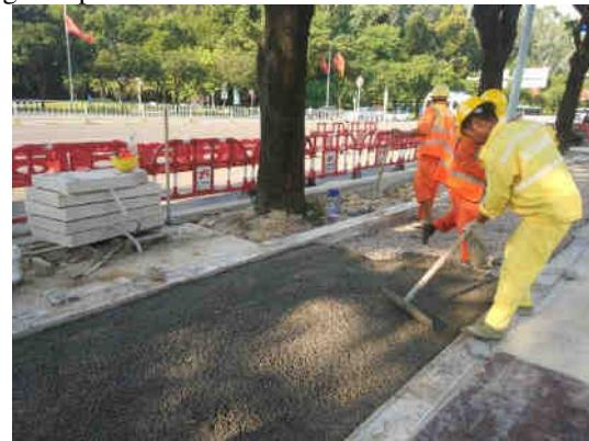
Fig.1 Permeable concrete paving
