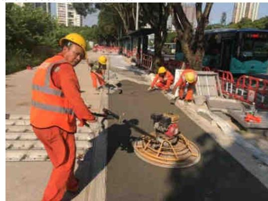
Fig.2 Polishing the surface
