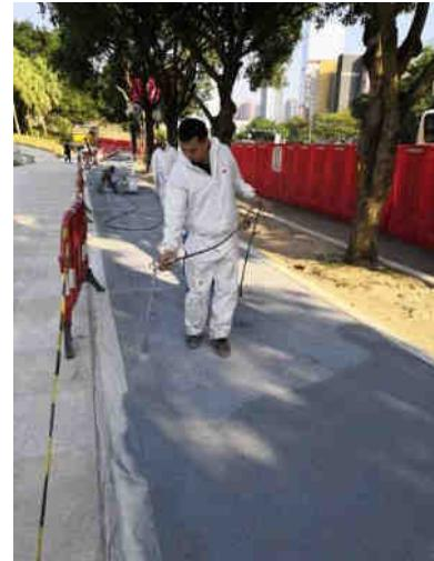
Fig.4 Spray sealant
