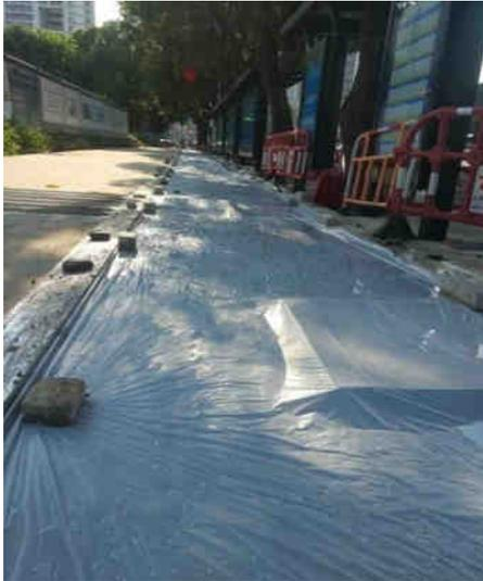
Fig.3 Film covering maintenance
