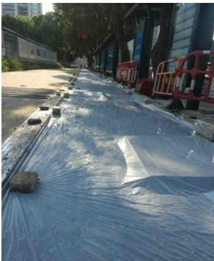
Fig.3 Film covering maintenance
