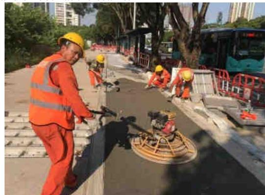
Fig.2 Polishing the surface
