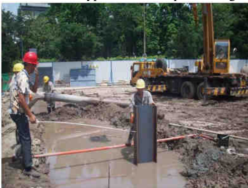
Fig. 6 measures the distance from the section steel to the positioning marker
