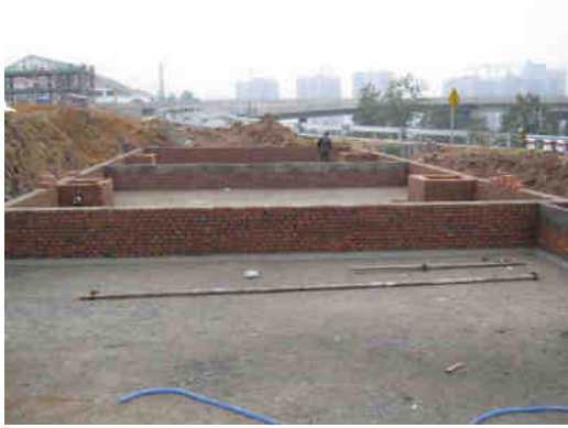
Fig.11 Construction of wetland bed body
