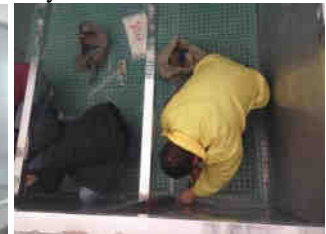
Fig. 7 Construction of the filter board
