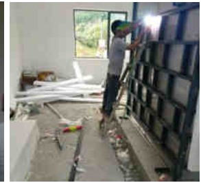
Fig. 12 Construction of the insulated outer wall
