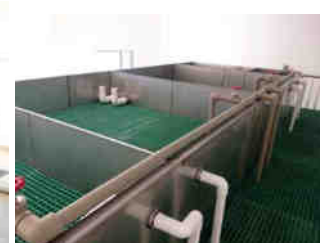
Fig. 12 Completed photo of the aeration biological filter 2
