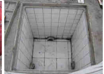
Fig. 6 Construction of the collecting pool
