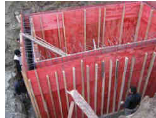
Fig. 5 Construction of the primary sedimentation tank
