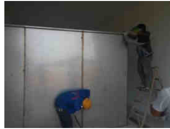
Fig.11 Construction of the sedimentation tank
