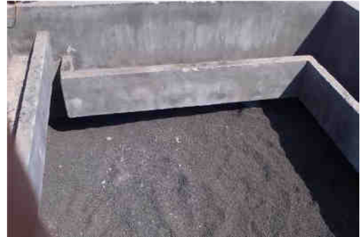
Fig.13 Wetland packing and fill
