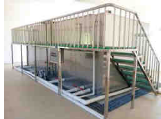
Fig.13 Aeration biological filter completed photo 1
