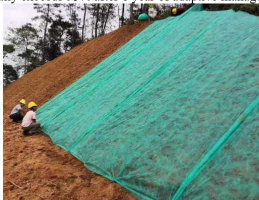
Figure.9 Post-Spraying Slope Coverage and Maintenance
