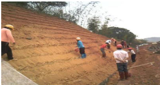
Figure.3 Slope Surface Preparation Operations
