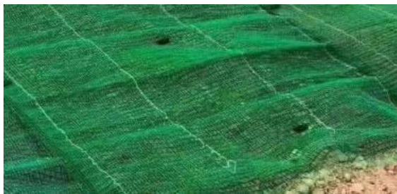
Figure.4 Three-Dimensional Mesh Installation Effects
