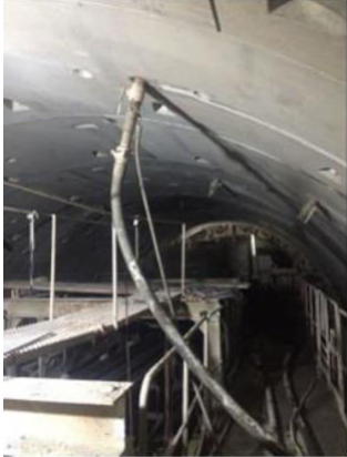
Fig.1 Secondary grouting after pipe segment wall
