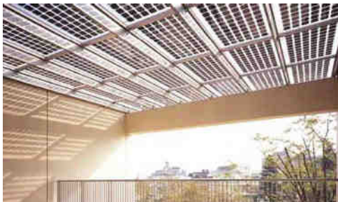
Fig 16: Image of a commercially available —light thrul BIPV Product.
