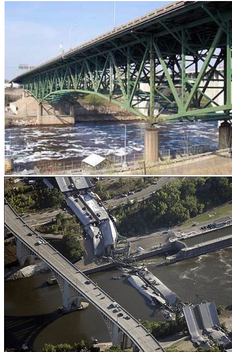
Figure . (Left) I-35W Bridge in Minneapolis, Minnesota; (right) catastrophic failure after collapse on August 1, 2007 (source: Associated Press, 2007).
