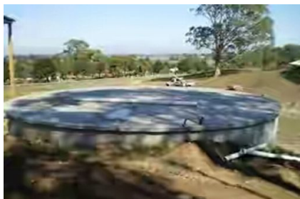
Fig. Under ground water tank
