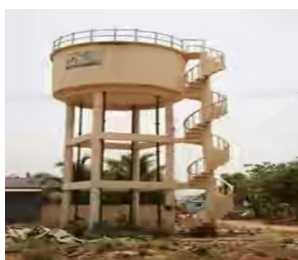
Fig. Elevated water tank
